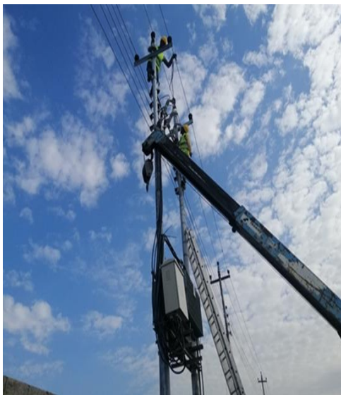
Transformers are installed and connected to the poles.
