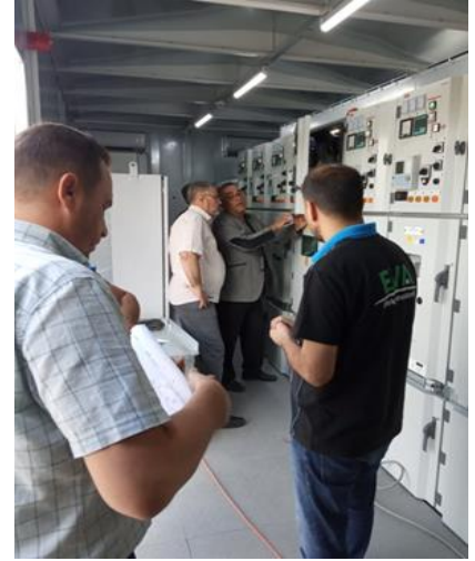
The factory test included, among others, testing the megger (left and centre) and the switchgear (right).
