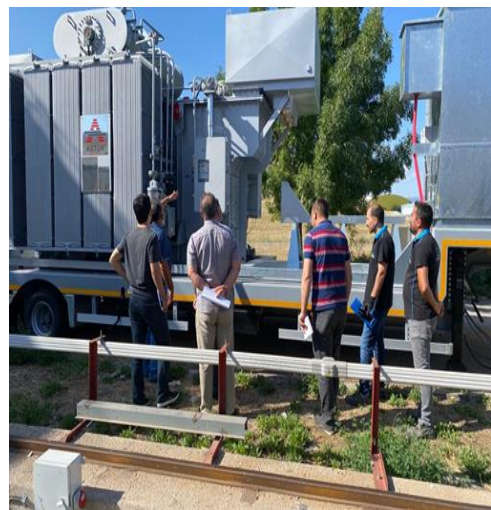
Visual inspections of the switchgear cabinet (left) and tap changer (right) were carried out.
