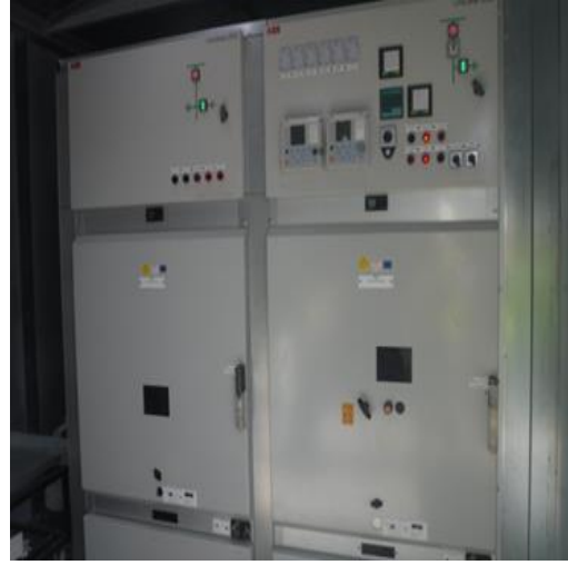
33Kva switch gear
